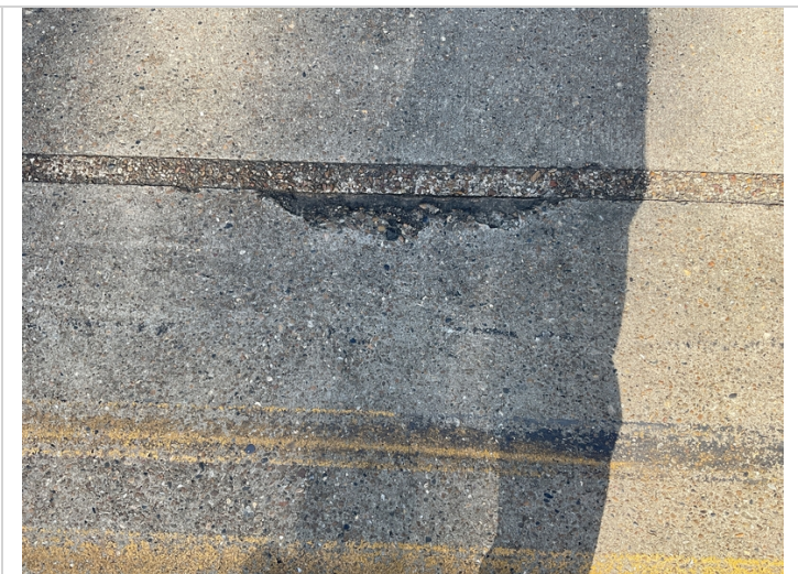
Minor delams in various locations
