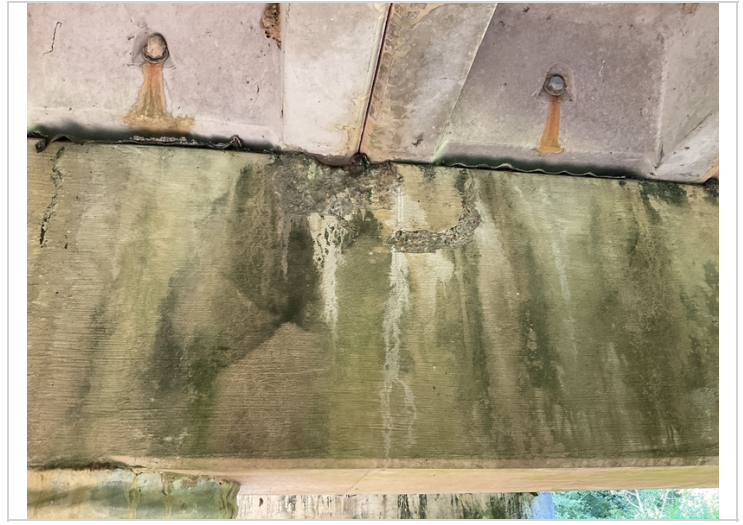
Spall bent 3 north face of cap
