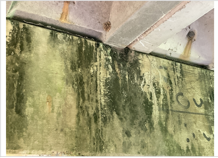
Spall bent 3 north face of cap
