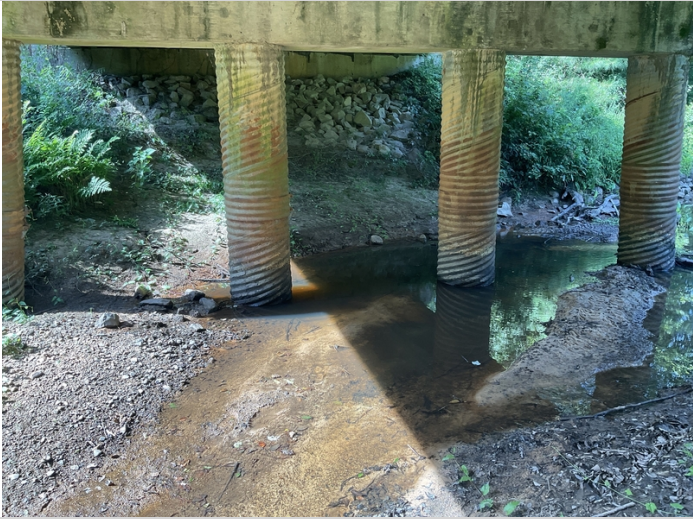
All piling have been encased by steel culvert pipe and beginning to show signs of corrosion
