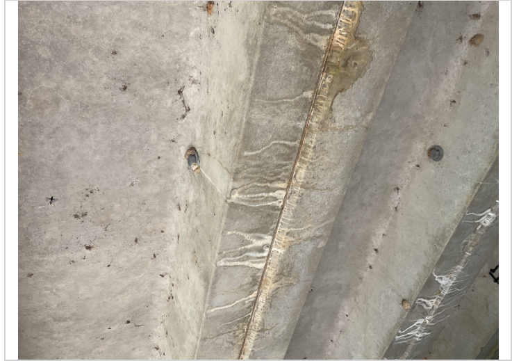
Salt leeching through all joints underside of deck
