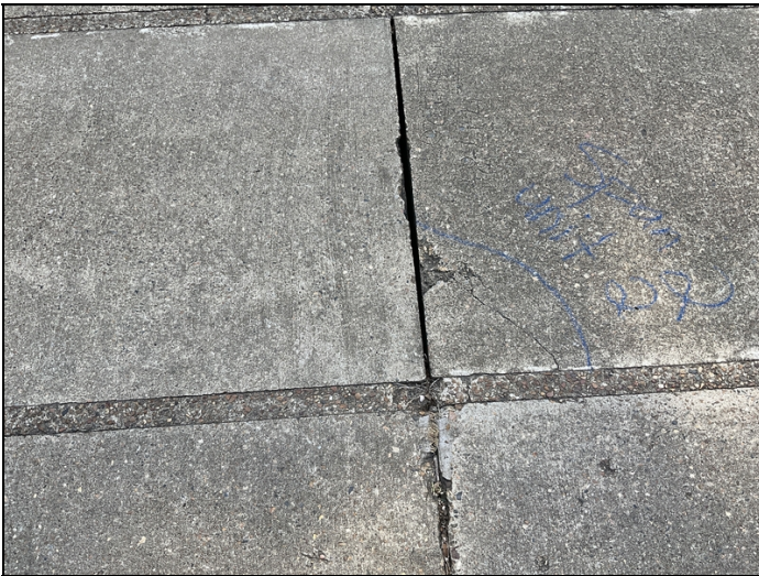
Joints need to be cleaned out from debris and reported back
