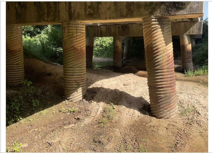
Scour hole beginning of bridge right side
