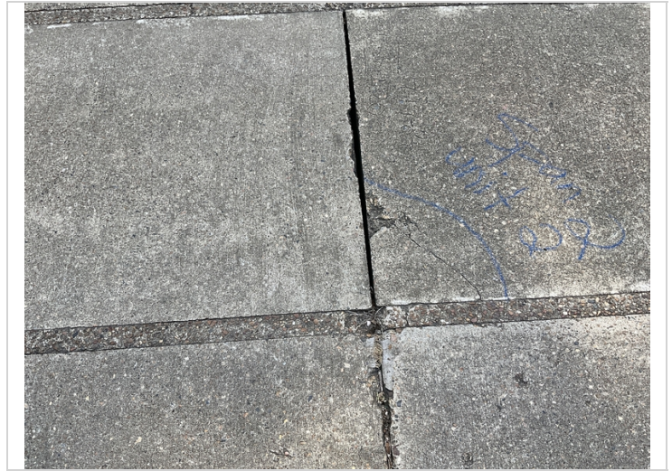
Joints need to be cleaned out from debris and reported back
