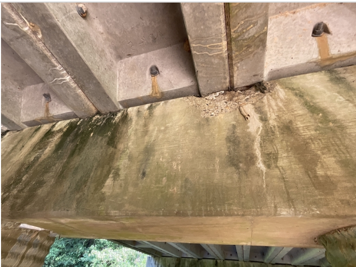
2 spall bent 3 cap south face
