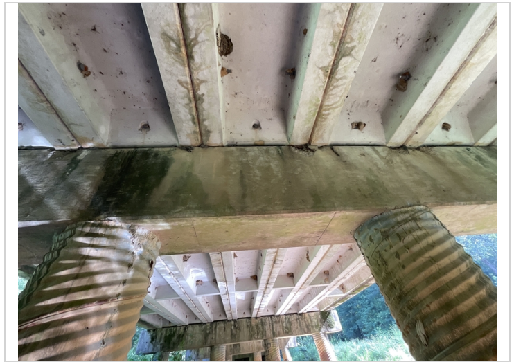
3 spalls on bent 5 cap south face
