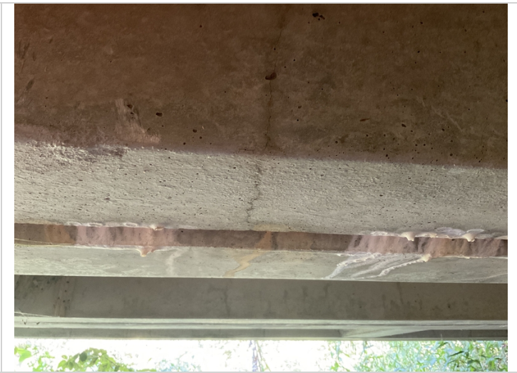
Minor cracking in various locations on underside of precast units
