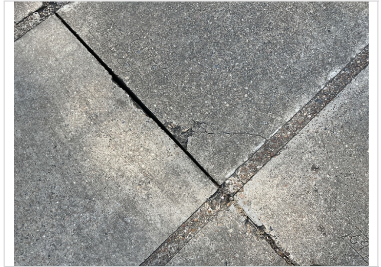
Some cracking in precast units various locations on deck
