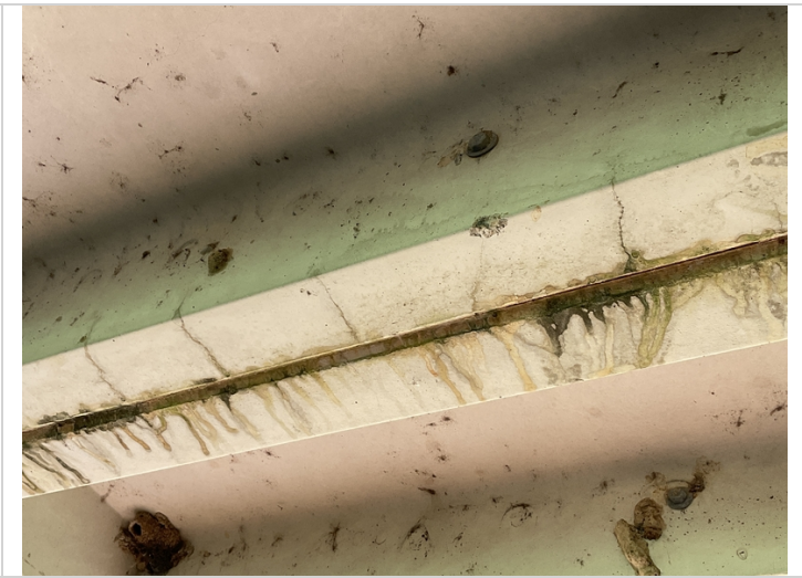
Cracks in bottom of precast units various locations of all spans
