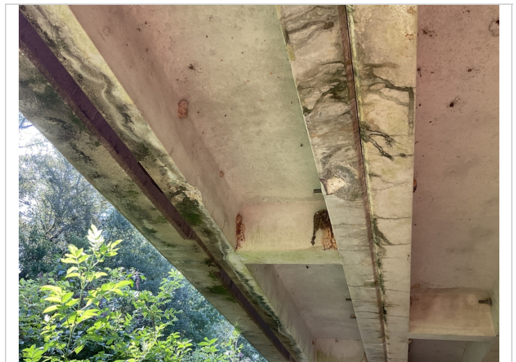
Span 5 unit 1 has two delams
